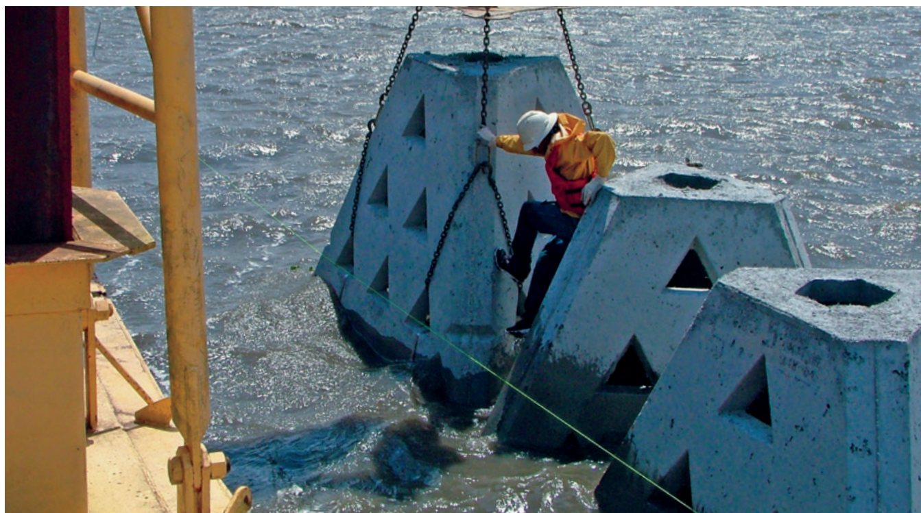
Wave attenuation device placement began at Lost Lake in May 2015.
