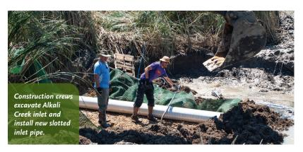
the wetland. Since then, waves eroded a small portion of the bank and sediment clogged the water control structure's inlet pipe. DU engineers added rock riprap to the eroded portion of the embankment and installed a new, slotted inlet pipe enveloped in engineered rock gradations to inhibit future clogging.
